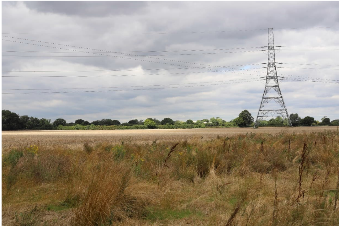
Plate 3: View Northwest From PRoW Sykehouse 29 Across Field SE2 included within the Southeast Part of the Solar PV Site
